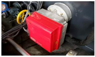
Complete unit equipped with 2 Italy Riello RG5S automatic burner and inner heating transfer oi boiler. Not need connect out boiler or heating.
